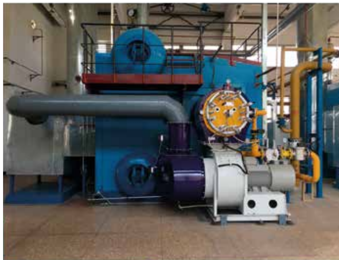
Beijing Aerospace University. Two 14MW Ultra Low NOx burner / 13ppm with FGR
