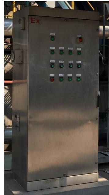
BMS Panel - Stainless Steel, Explosion Proof With Internal Air Purge System
