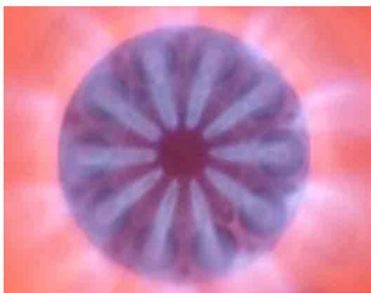
FIGURE 4 – TYPICAL ULTRA LOW NO x BURNER FLAME USING FGR
